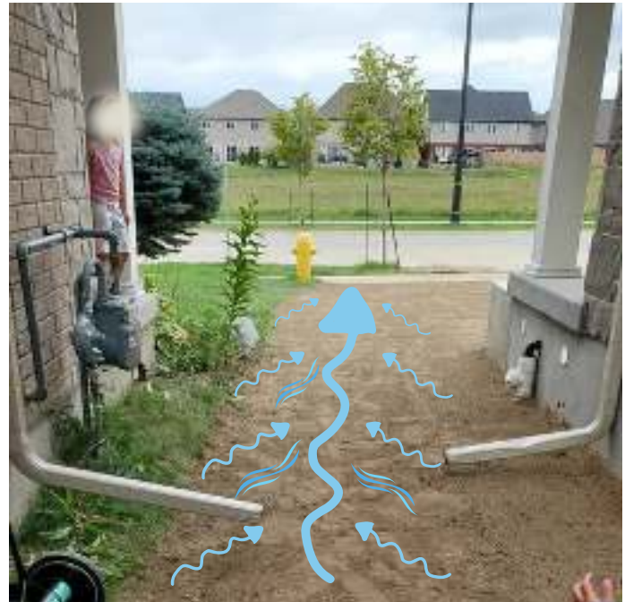
Swales are often located between homes. When planning a garden next to your neighbour's property, care must be taken to NOT alter the slope as it can affect water drainage Image: Reddit for Landscapers
